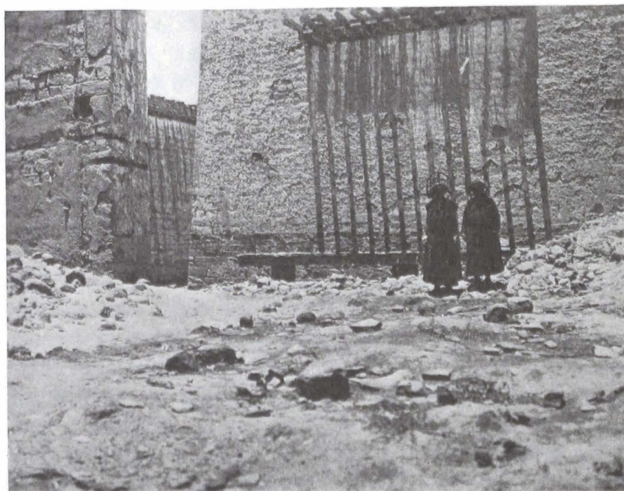
The granary at Palha (right). Note the ventilation holes at the base of the wall
